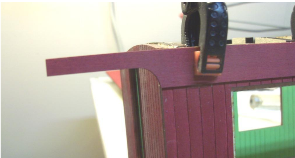
I used a rafter to help clamp on the 4 windows side.
