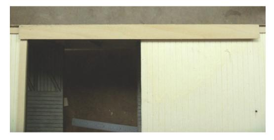
Remove the door, lower door glides and door stop and repeat for the other side door.
