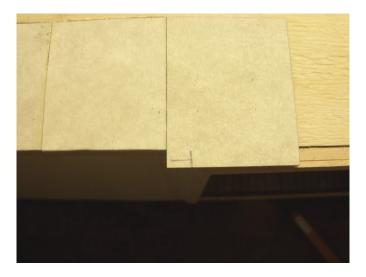
This tile gets a corner snipped and a part bent down. The ends over the door don't get bent down.
