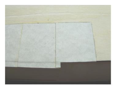
Mark and cut the last tile as needed and glue down. Any spacing issues will be covered by the catwalk end platform.
