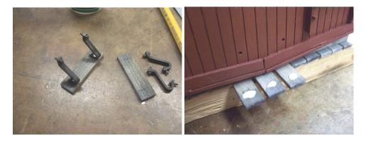
Add a drop of ACC to the support tips and position the supports into the holes and push the board into position as pictured.
